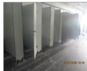
Photo of the sanitary facilities Toilet.JPG
